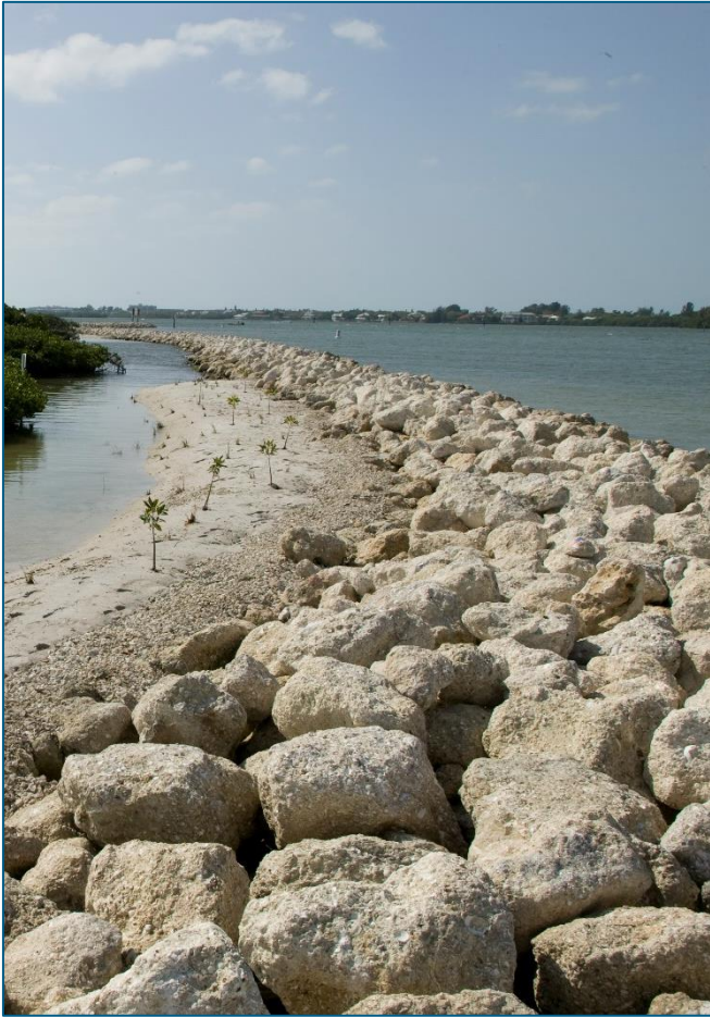
Breakwater with vegetative plantings
