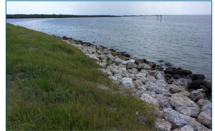
One year after construction
