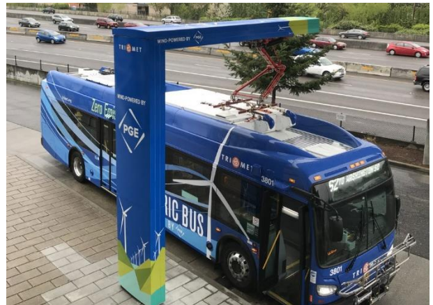
“A Portland, Oregon TriMet Battery Electric Bus Charging”
