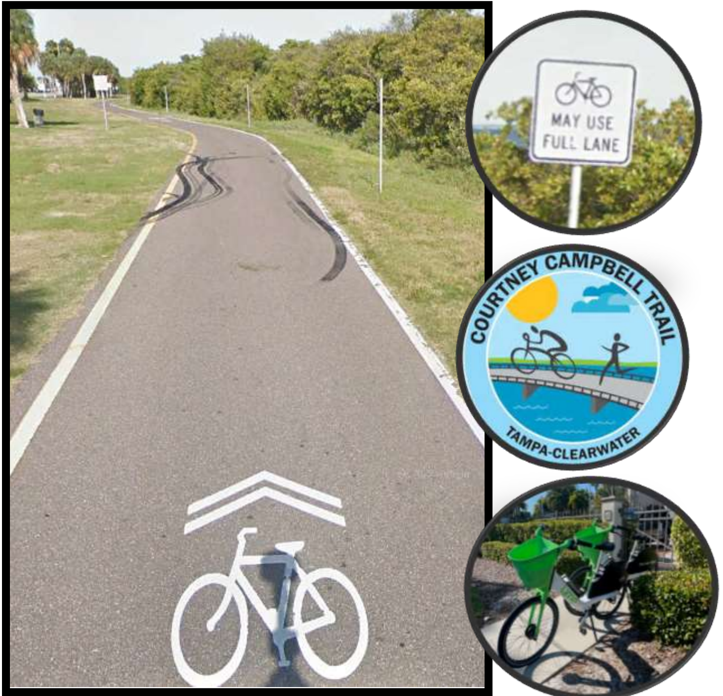
Figure 6, Public Safety & Environmental Concerns – Roadway Safety
