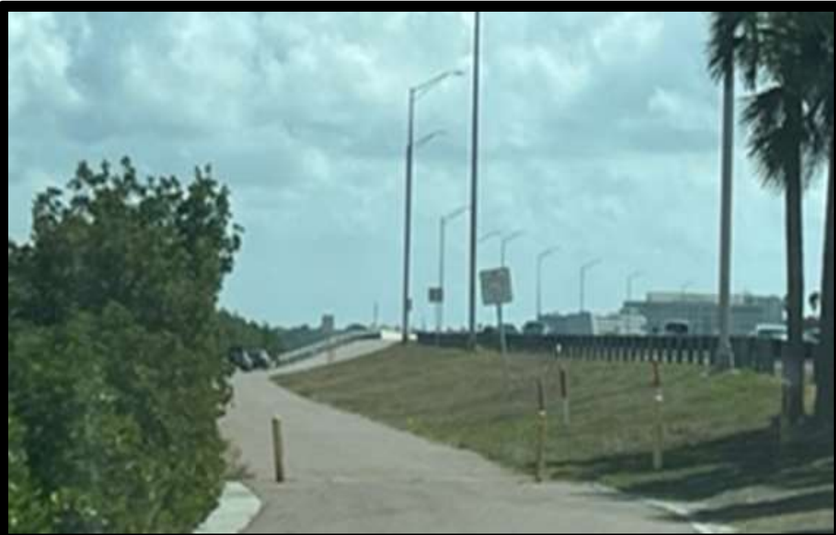
Figure 8, Public Safety & Environmental Concerns – Direct Access to the Virginia Creighton Bridge
