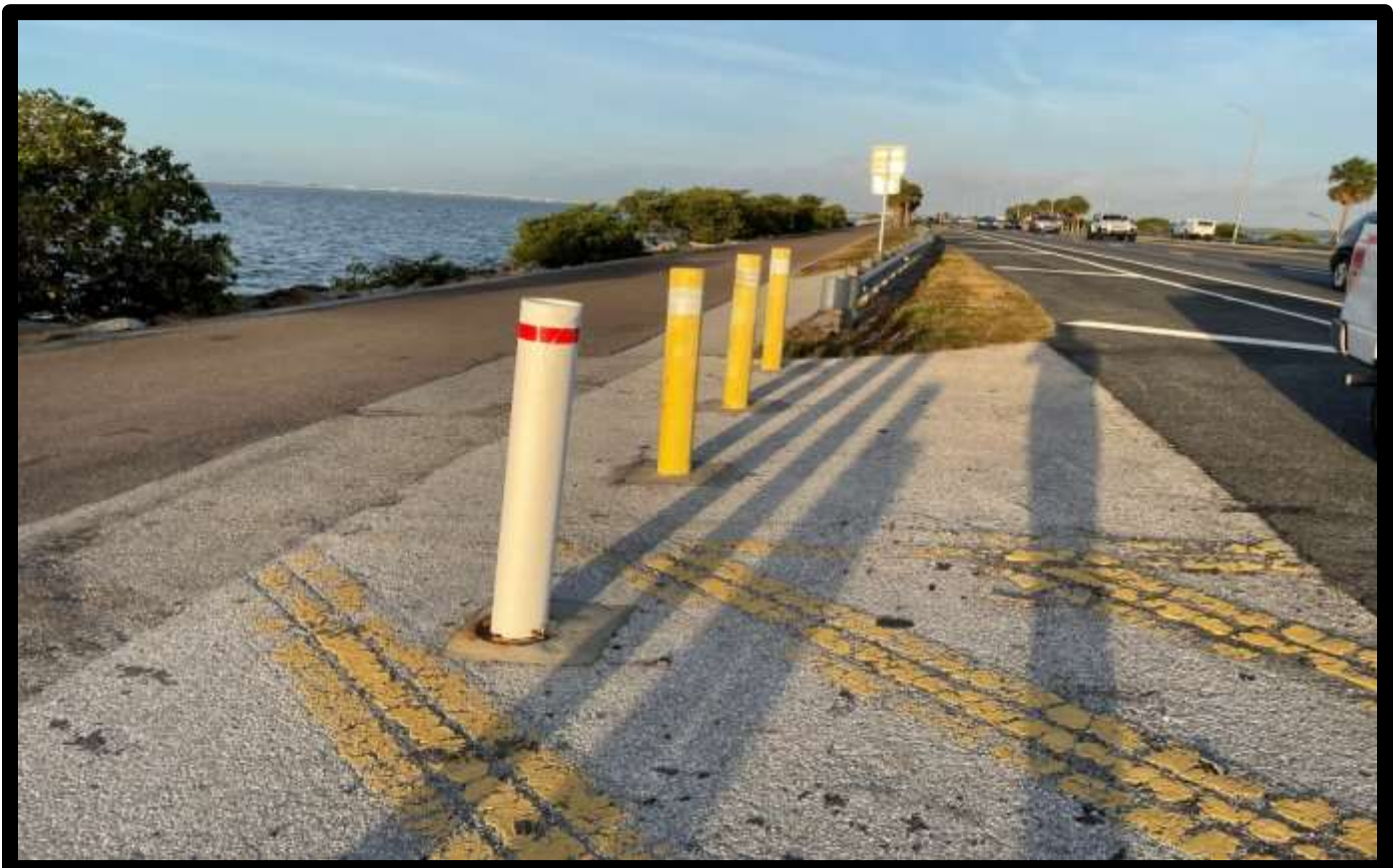
Figure 13, Bollards Providing Vehicles Trail Access from the Hwy. in Pinellas
