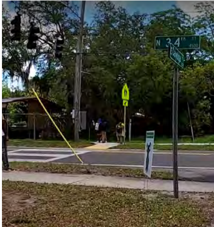
Image 19: Pedestrian Hybrid Beacon on N 34th Street
