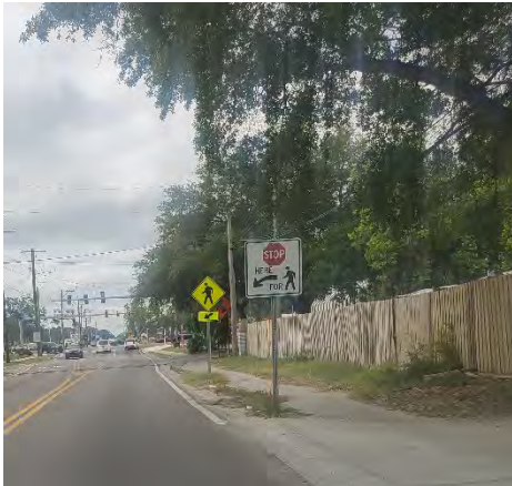
Image 12: Crosswalk Signage where Crosswalk is not Present
