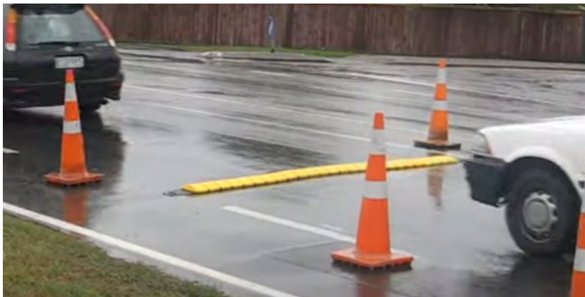
Image 6: Portable Speed Bumps
