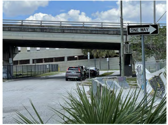
Image 63: Narrow Pedestrian Walkway and People Parking where Parking is Prohibited
