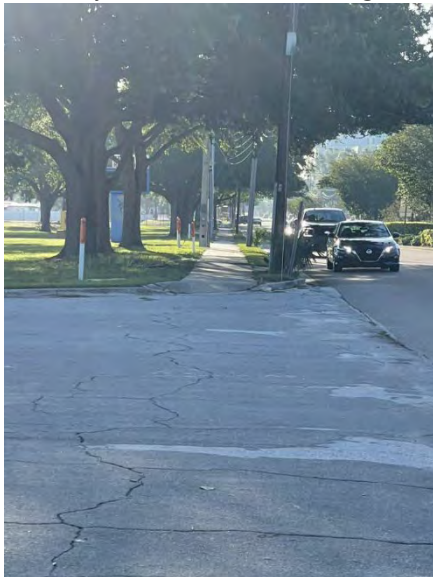
Image 51: Width of Exit of School Loop at W Cypress Street
