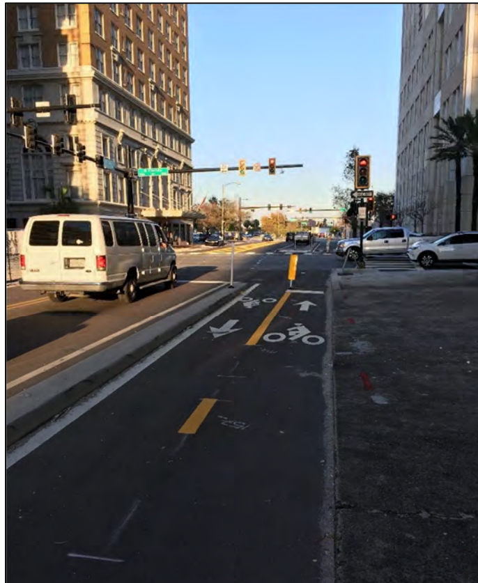
Figure 3.8 Cycle track on East Cass Street, Tampa, FL.
