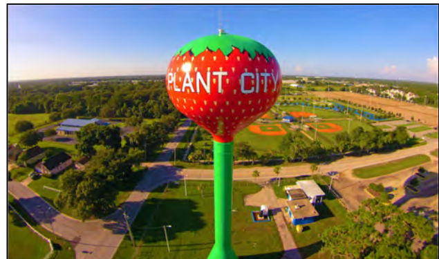
Plant City Water Tower. Source: Plant City Observer.
