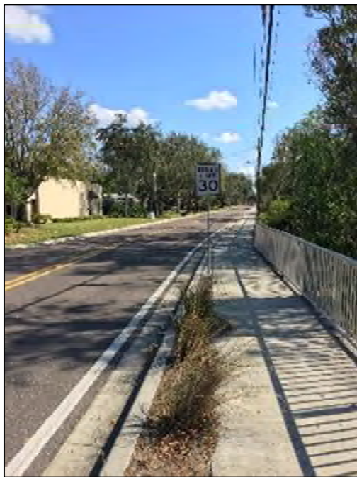
Figure 2.1 Mendonsa Road sidewalk. Source: Project Team.
