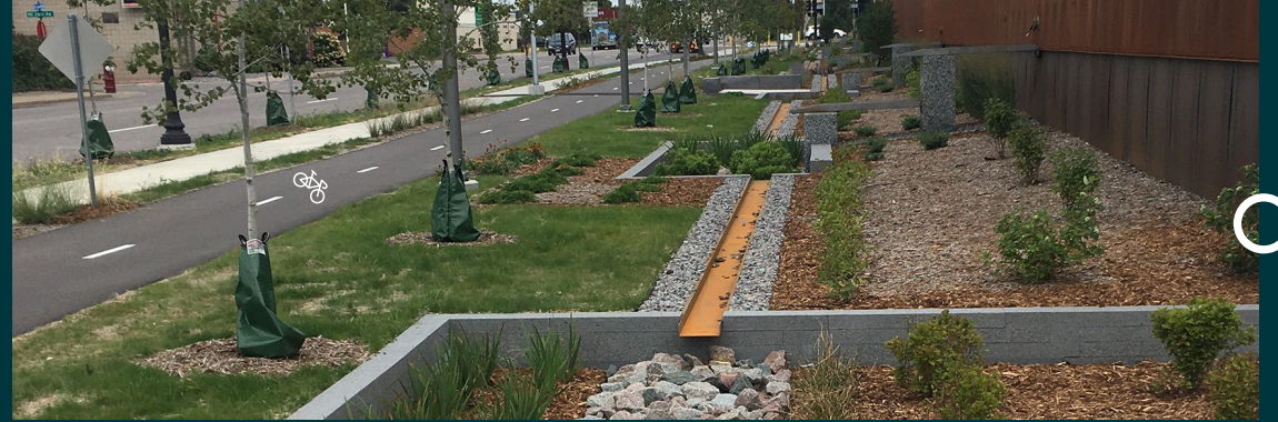
Complete Street Features & Enhanced Stormwater Facilities
