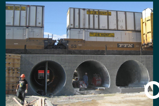
Strengthened/ Enlarged Culvert Structure
