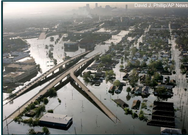
Within the top image, sections of Interstate 10 are underwater in the City of New Orleans post Hurricane Katrina.
